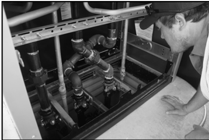
New Requirement - Installation of under-dispenser containment (UDC) for all new or replaced dispenser systems
