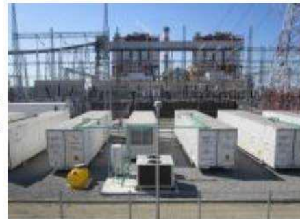
5 MWh A123 battery in Chile
